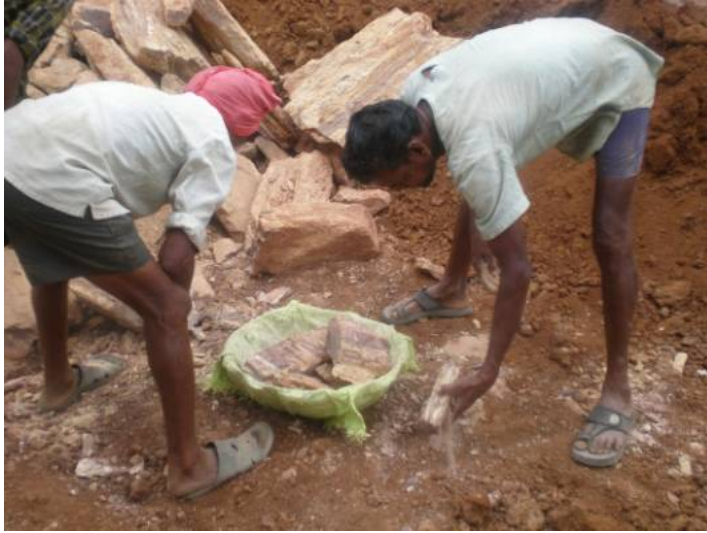
Breaking and moving the stone for the foundation.
