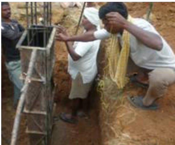
The 'trench' foundation is made, next the Pillar is made – cast.
