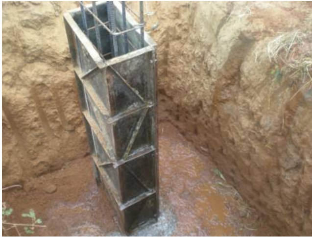
The 'trench' foundation is made, next the Pillar is made – cast.
